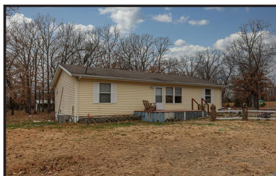
3BR, 2BA TRUMAN LAKE HOME on 20 +/- acres on blacktop road. Newer septic system. 30x550 shop. Home is minutes away from lake access to Truman Lake. Property also has 2 RV hook-ups. Trail road gives you access to back of the property. Lots of wildlife. $270,000 Call Jennie today! MLS#96634
